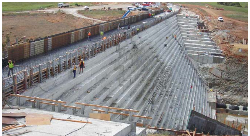
North Para Flood Control Dam, September 2007
